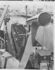
LIKE A mother hen and her chickens, the Queen of Holland begins dredging operations, above, in San Nicolas Harbor. This bridge work, right, supports the ladder which houses the cutter mechanism. MANERA UN gainja cu su poctionan, Queen of Holland ta cuminza draga, ariba, den haaf di San Nicolas. E puente, banda drecha, ta wanta e trapu cu ta hospeda e mecanismo di cortá.
